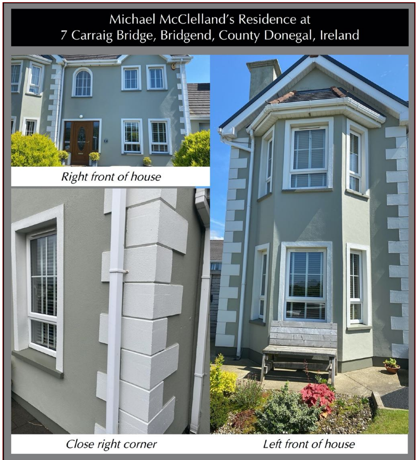
Figure 1: Field photos of the home from different sides showing the overall sound condition of walls and the absence of any visible cracking.
