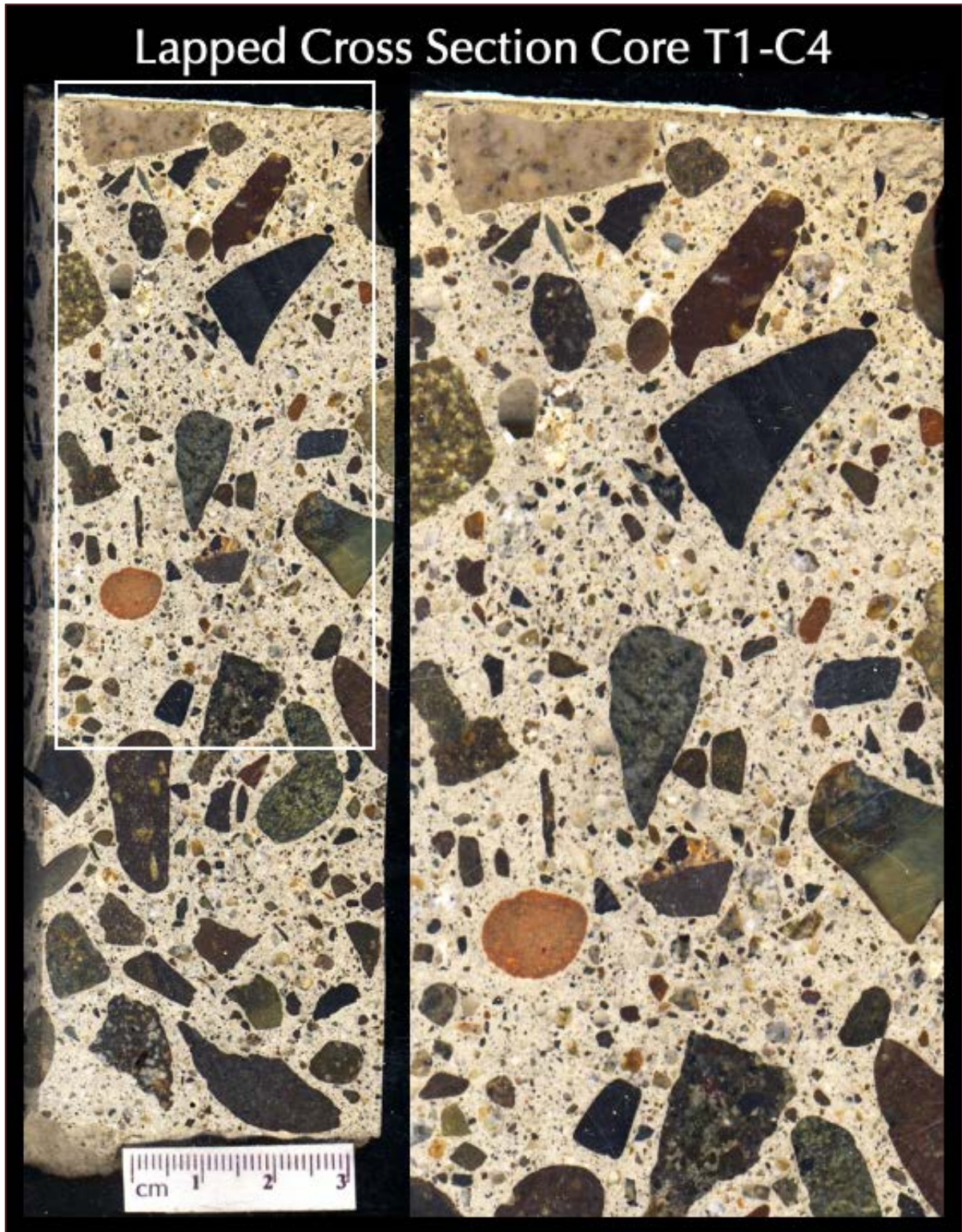
Figure 17: Lapped cross section of Core T1-C4 showing: (a) a thin paint coat at the top well-bonded to the underlying concrete having a nominal thickness of < 1 mm; (b) the main concrete body containing crushed volcanic and volcaniclastic gravel coarse aggregate where aggregate particles are subrounded to subangular, dense, variably colored, well-graded, and well-distributed, natural siliceous sand and finer fractions of volcanic rocks and minerals in fine aggregate, all dispersed in a Portland cement paste; and, (c) the overall sound (visually crack-free), dense, well-consolidated nature of the concrete in the body. The boxed area at left is enlarged at right.
