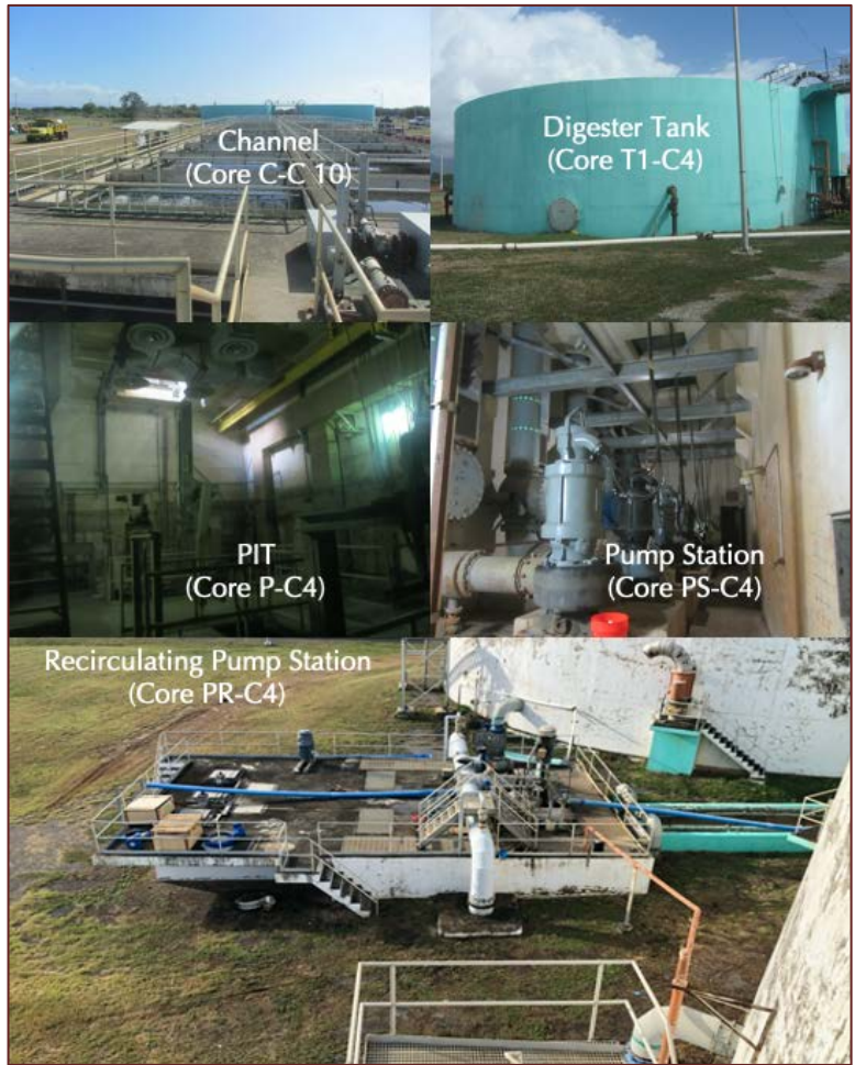
Figure 1: Field photos of five structural elements of wastewater treatment plant from where five concrete cores for this study were reportedly retrieved. The core ID received for each structure is marked.
