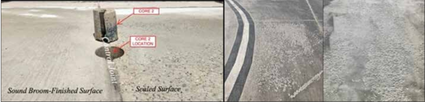
Case 3: Scaling in Type IL + SCM (35% slag), w/cm 0.45, 7% air, 3500 psi mixture Slab-on-ground, Michigan, USA
