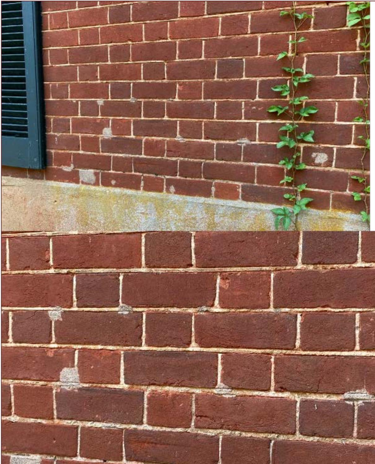
Figure 2: Brick masonry wall of courthouse from where mortar sample for this work was, reportedly, collected. The bottom photo is an enlarged view of the central portion of wall from the top.
