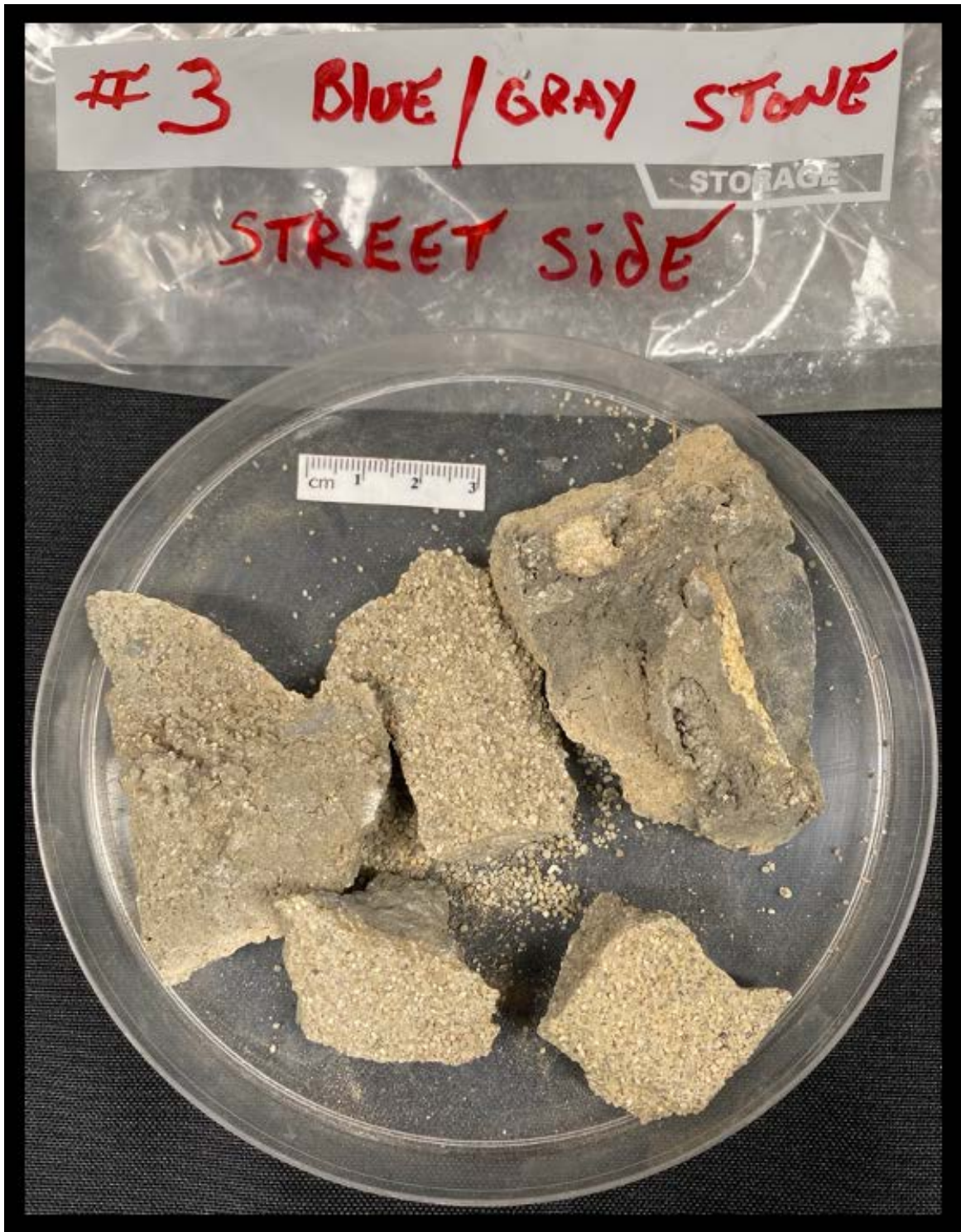
Figure 3: Mortar fragments #3 marked as 'Blue/Gray Stone Street side '(hereafter described throughout the report as Mortar #3). The sample consists of several rectangular pieces from the mortar joint that are mostly weathered brown to dark gray with excessively sand-textured exposed faces. Overall integrity of the pieces is moderately hard, in fact noticeably harder than typical historic lime mortar suggesting the potential presence of a Portland cement based component in the binder, which is responsible for the dense hard medium gray nature of fresh fractured surfaces of pieces. Notice loose sand particles on the faces that have been plucked out from the fragments during recovery.
