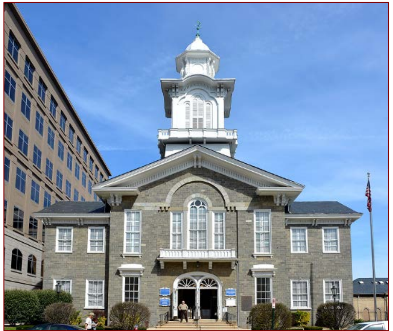
Old Lehigh County Courthouse 455 Hamilton Street Allentown, PA
