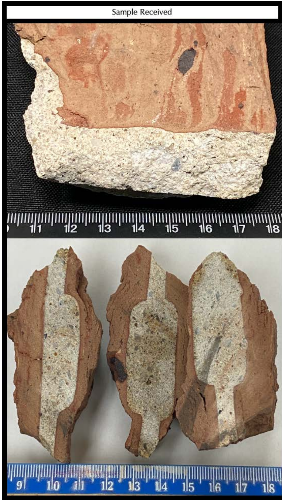
Figure 5: Additional photos of the solid chunk of a jointing mortar sandwiched between remains of brick masonry units where the mortar is exposed after sectioning the chunk into three pieces as shown in the bottom photo. Notice good bond between the brick remains and interstitial medium beige gray mortar.
