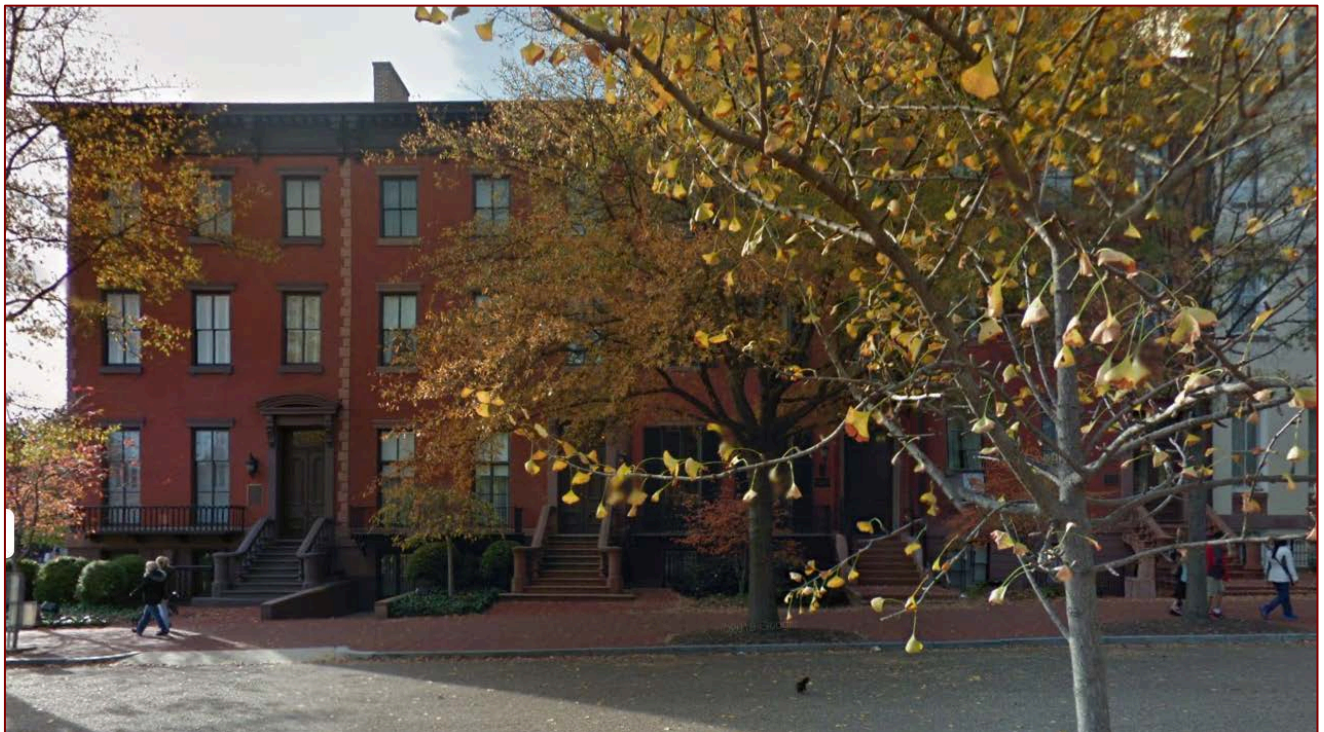
Figure 1: The building at 708 Jackson Place in Washington, D.C., from where three mortar samples were provided for detailed laboratory investigations.
