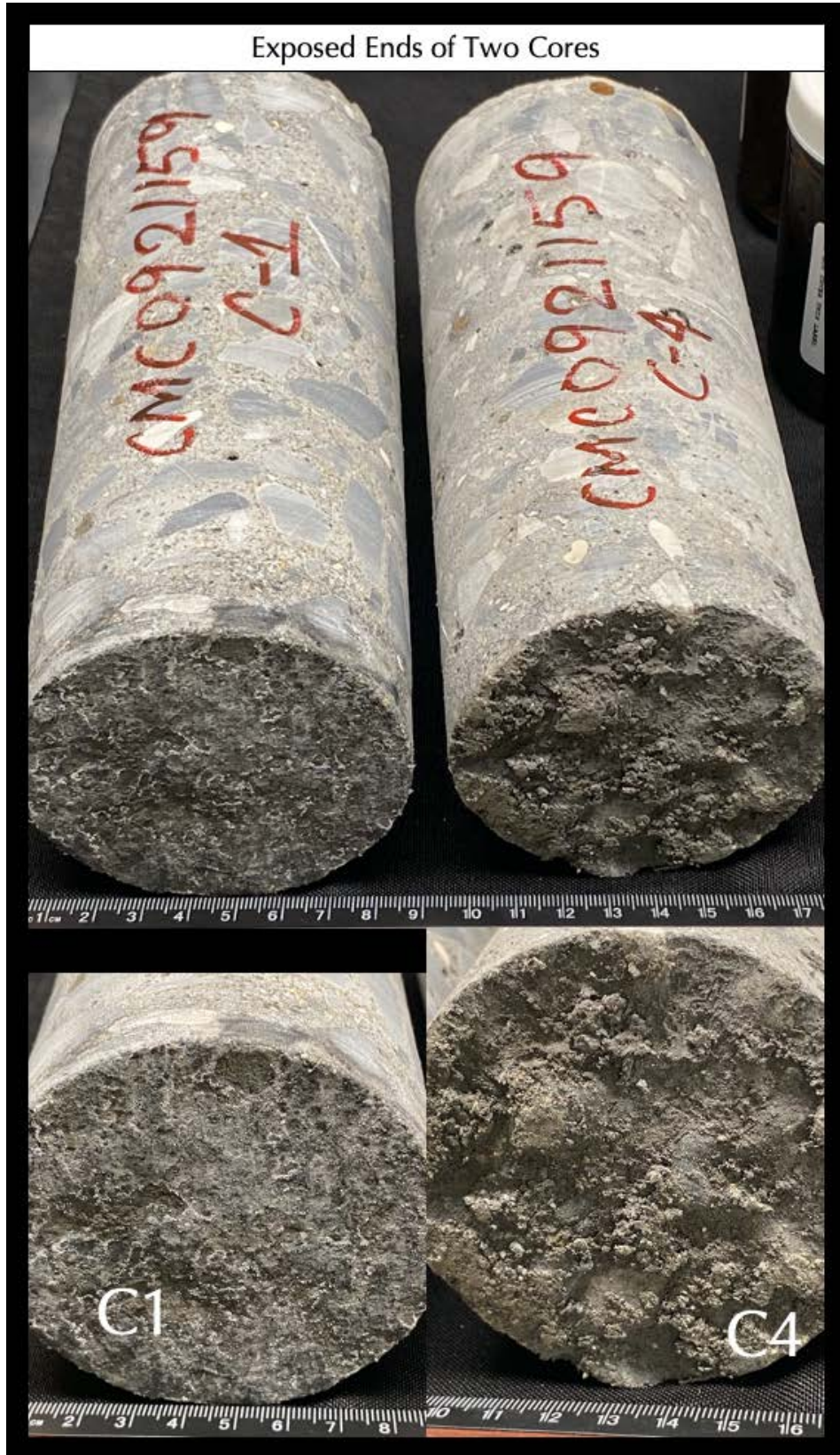
Figure 6: End surface (exposed ends) of Cores C1 and C4, as received, showing rough surfaces where Core C1 has a near-surface 'incipient delamination' present as elongated separations or 'tears,' whereas C4 has no such near-surface separations, but the entire exposed surface is rough.
