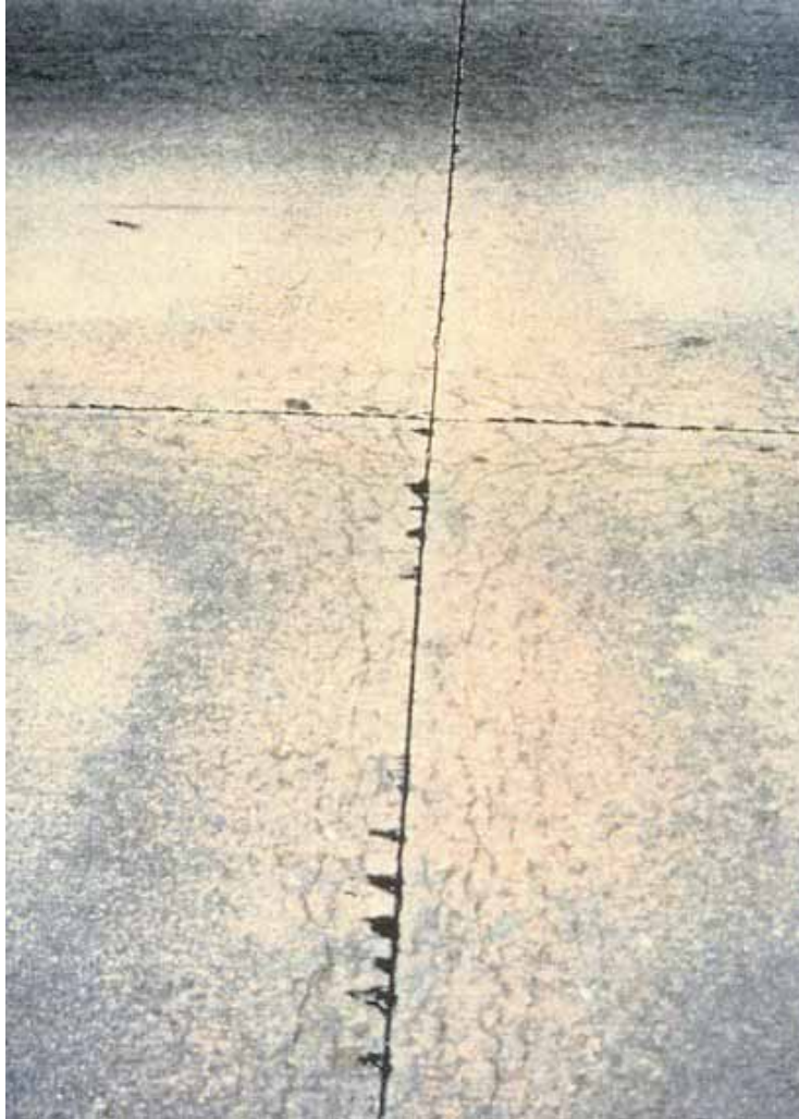
Figure 221. D-cracking of a pavement caused by destruction of the aggregate by cycles of freezing and thawing (cracking parallel to the joint and wrapping around at the juncture of joints defines D-cracking).
