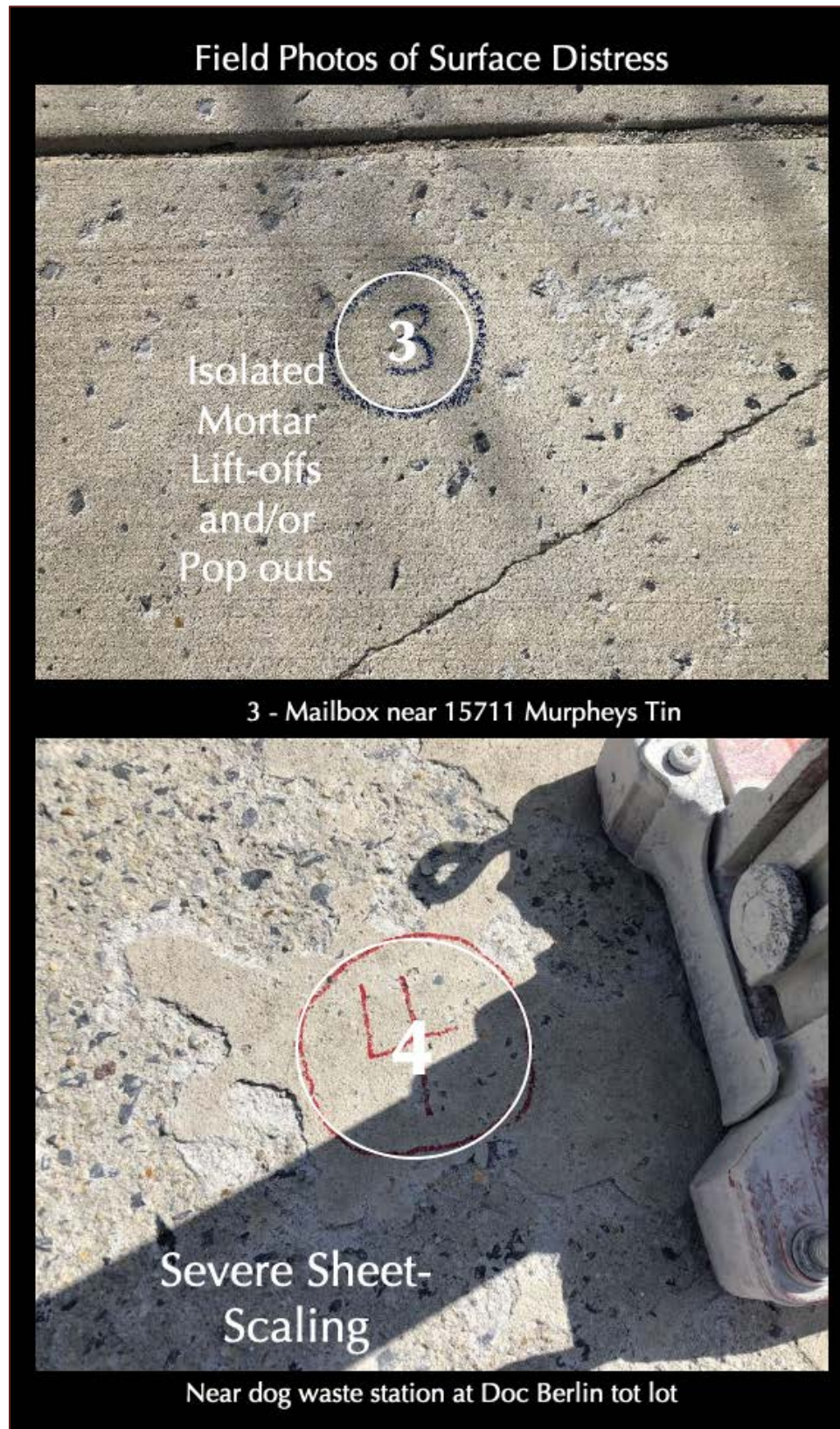
Figure 5: Isolated occurrences of surface distress as exposures of near-surface coarse aggregate particles as mortar lift-offs and/or pop-outs at the location of Core 3, but severe sheet-style surface scaling due to accumulation of bleed water underneath prematurely finished surface at the location of Core 4.
