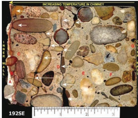
Fig. 4: Section of a core showing the extent of damage in the wall of a concrete chimney
