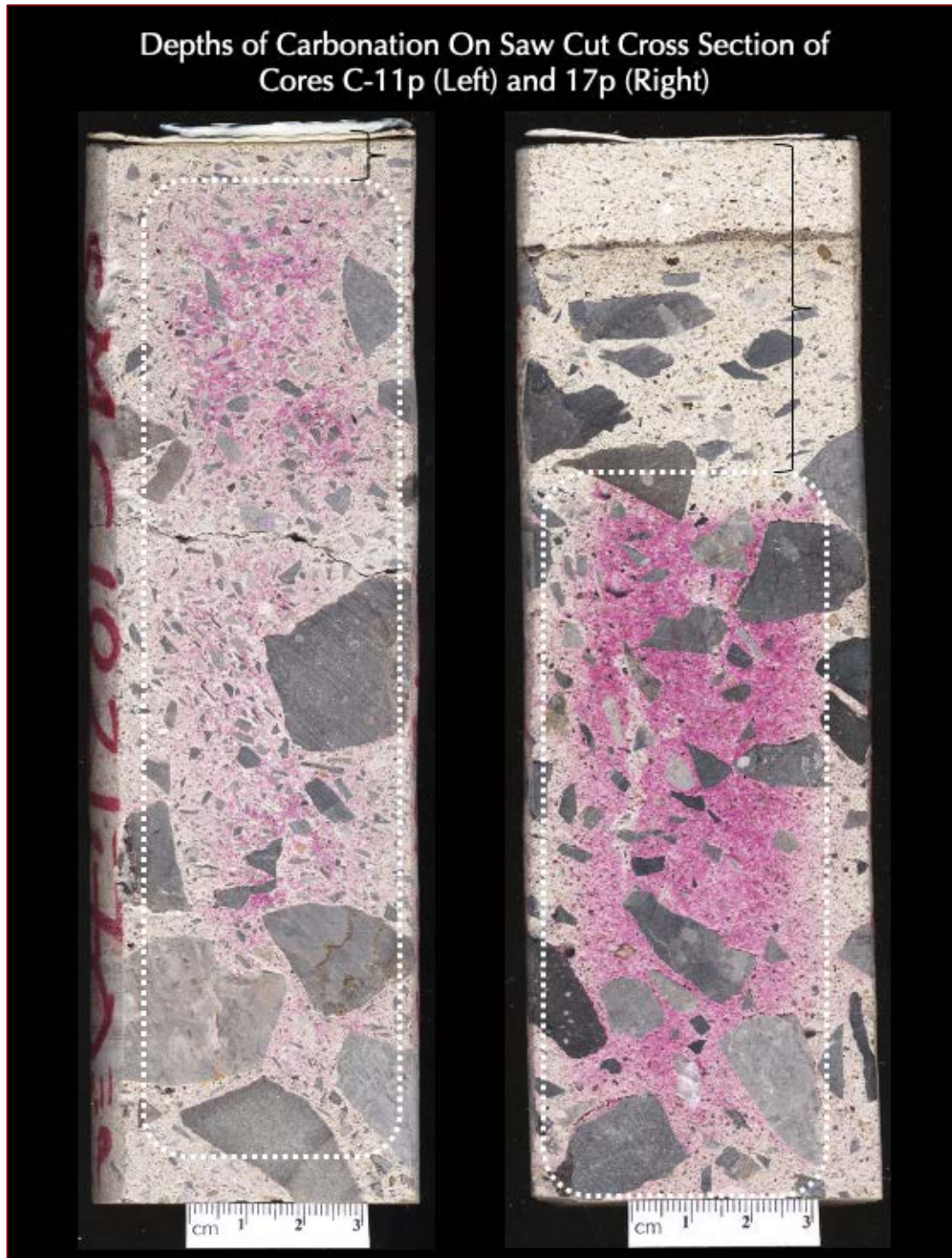
Figure 11: Saw-cut cross sections of Core C-11p (left) and C-17p (right) after treatment with phenolphthalein alcoholic solutions to show significantly deeper depth of carbonation of concrete in Core C-17p at right, which is measured to be approximately 40 mm after which the remaining 170 mm of concrete is non-carbonated and discolored to pink tone. Core C-11p, on the other hand, shows only a shallow depth of carbonation at the exposed surface region measured to be approximately 10 mm, after which the remainder of the concrete shows sporadic patchy carbonation due to inherent porous and permeable nature of concrete to atmospheric carbon dioxide. Boxed areas in both cross sections show interior non-carbonated or less carbonated concrete that have turned pink compared to carbonated surface regions that remained light gray after treatment with phenolphthalein solutions.
